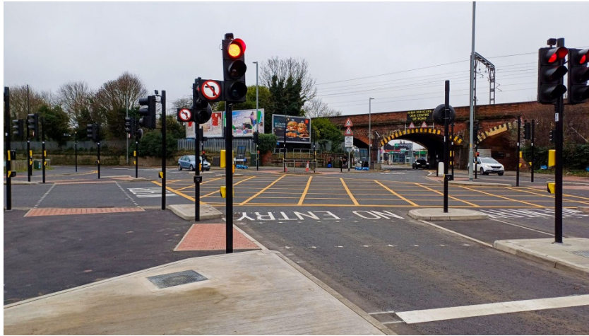
Station Road/ A607 Junction - 16 December 2024
