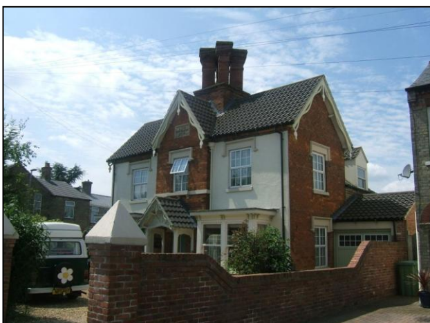
Fig.26 No.65 North Road, with attractive Victorian detailing such as decorative bargeboards, hooded moulds and diamond shaped chimneys.
