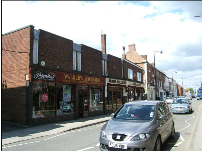
Fig.9 Post War developments such as 19 -23 North Street have a negative impact on the conservation area.
