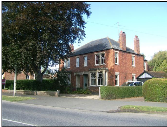
Fig. 29 No.12-14 West Road; an attractive late Edwardian property with refined features.
