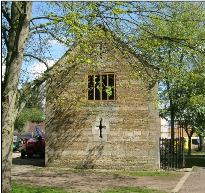
Fig. 20 Grade II listed Shippon Barn with arrow slits believed to have been part of the original Bourne Castle.
