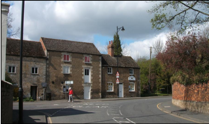
Fig. 13 The gentle curving character of South Street with Baldocks Mill directly addressing the Street and an attractive boundary wall to No.32 on the right.
