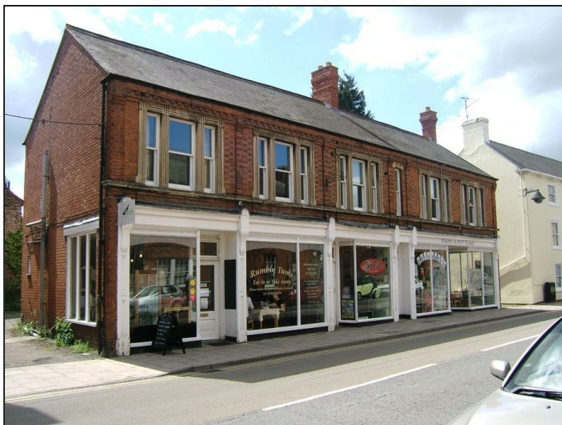
Fig.11 Buildings that retain their traditional shop fronts such as Nos. 25-31 above make a positive contribution to the character of West Street.
