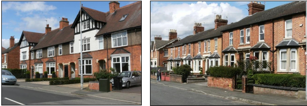
Front gardens converted to off-street parking have a negative impact on street scene
