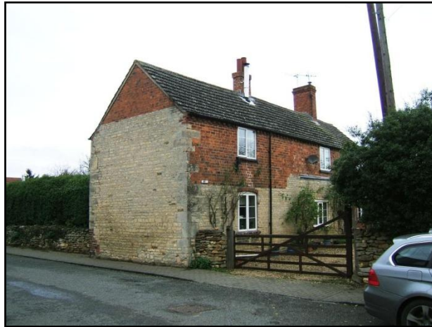
Fig.3 The combination of Random rubble stone and brickwork is a common vernacular approach used across the conservation area.
