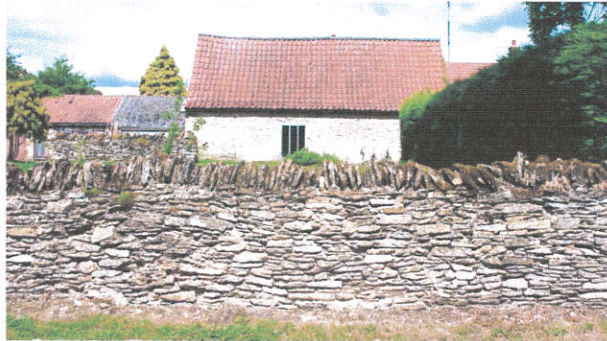
Dry stone walls, a feature of the village
