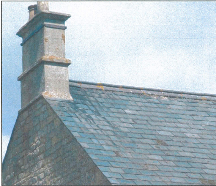
◀ Slate roof and stone chimney of former Pub
