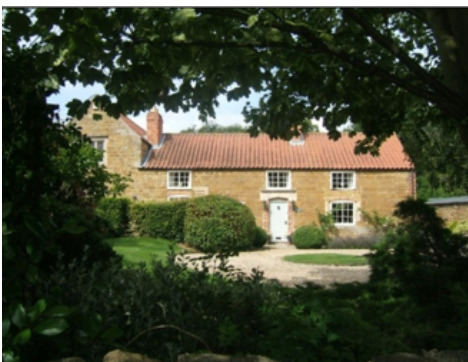
Fig.8 Grade II listed Plum Tree Cottage; built of harmonious material palette of ironstone with red pantile roof
