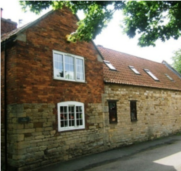
Fig.12 The Old Stables, The Green with an L shaped plan form and an attractive mix of coursed limestone and brick.
