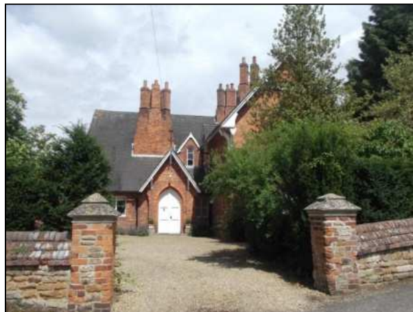
Fig.15 The Old Vicarage, clearly displaying features typical of the Brownlow style such as the triple twisted chimneys, prominent gables and fretted bargeboards.
