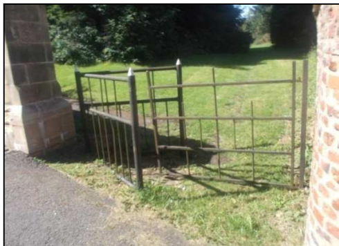
Fig.11 Cast iron gates located along the footpath that runs between the Church and Low Road are an attractive feature and should be retained.
