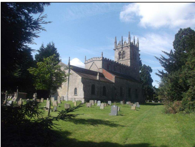
Fig.2 Church of All Saints (Grade I) together with the motte and Bailey form areas of visual dominance and high heritage significance. The church is located within a spacious cemetery with mature trees such as yews framing views.
