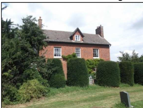
Fig.14 Church Farm, encloses the churchyard at its northern end, to the rear of the property is a panoramic view of the Vale.
