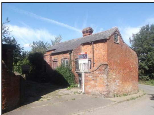
Fig.16 Outbuildings at The Cottage, display an exuberant style with decorative chimney stacks, typical of the design found within the 'Brownlow' estate.
