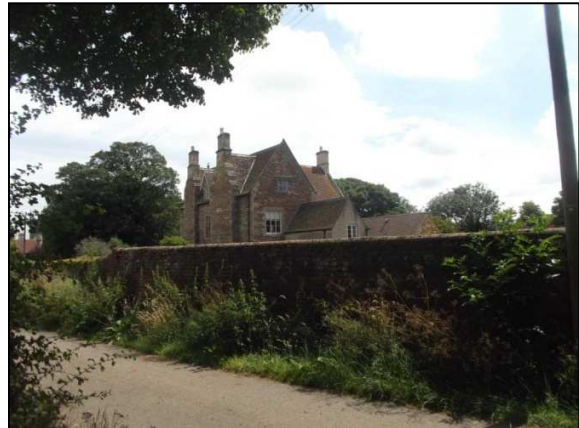
Fig.5 Hough Manor (Grade II), with tall boundary wall partly obscuring its view. The building, together with its grounds to the front and rear, and enclosing boundary walls make a significant contribution to the conservation area.
