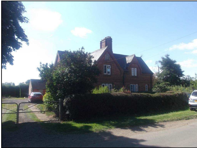
Fig.1 Nos.29 and 30 Frieston Road; typical of the 'Brownlow Estate' type with prominent gables, twisted chimneys and a hedgerow to the front boundary.
