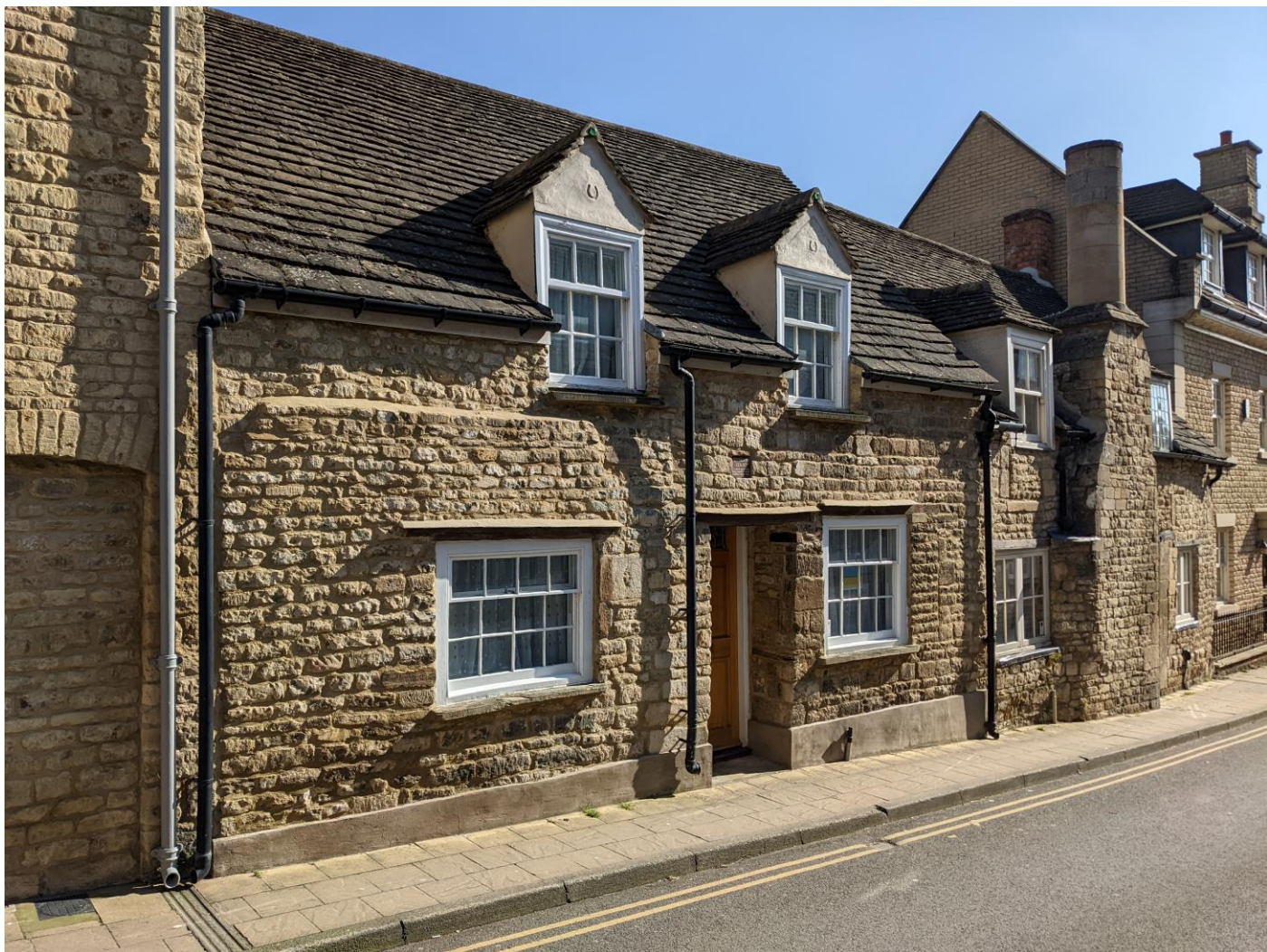
Frontage 9-10 St Georges Street, Photo taken 10 th March 2022
