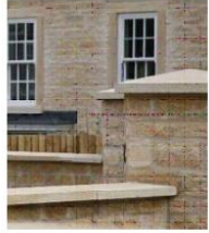
Proposed stamford masonry coping stones to be used
