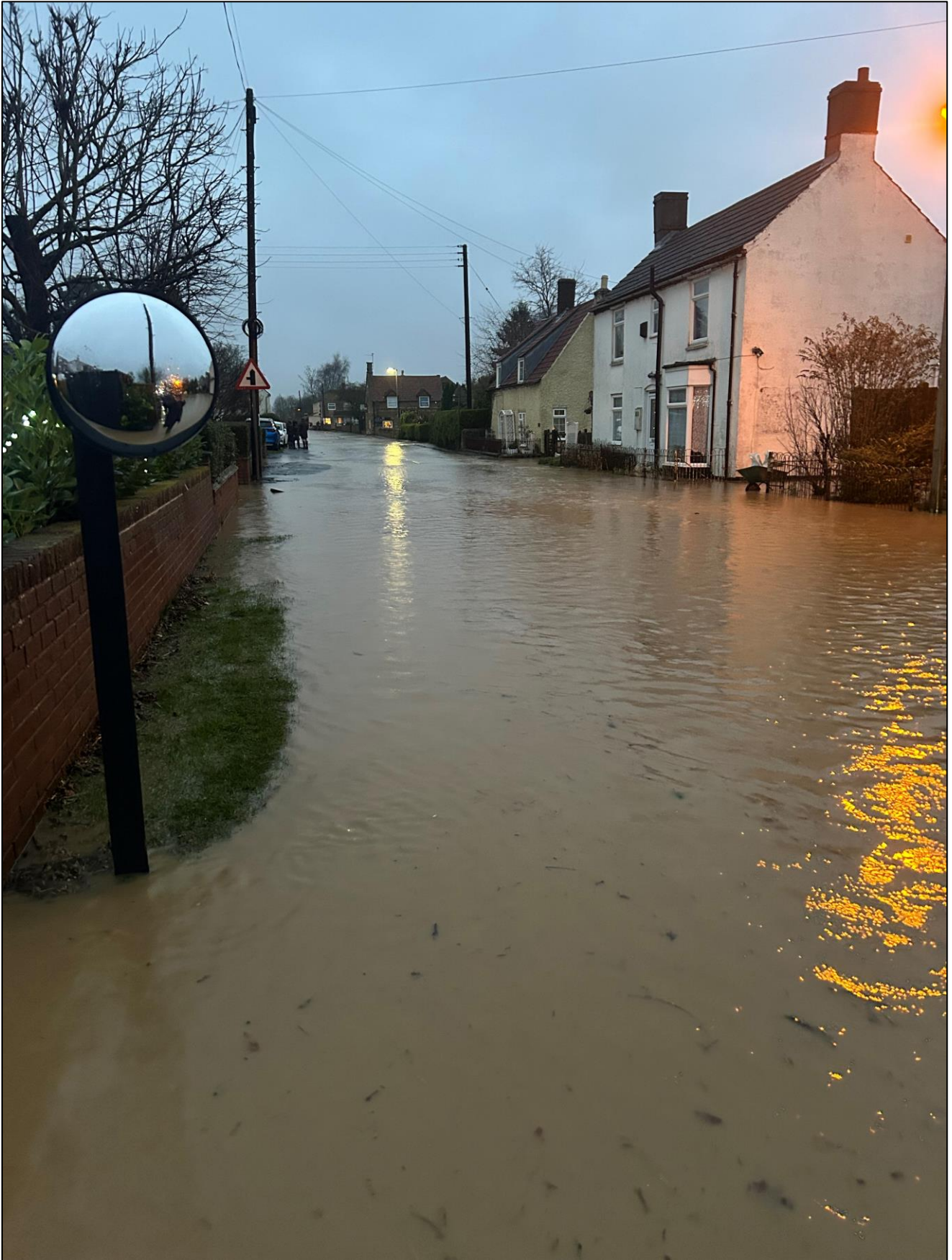
(Photo 3 – External flooding during Storm Henk in Pointon)
