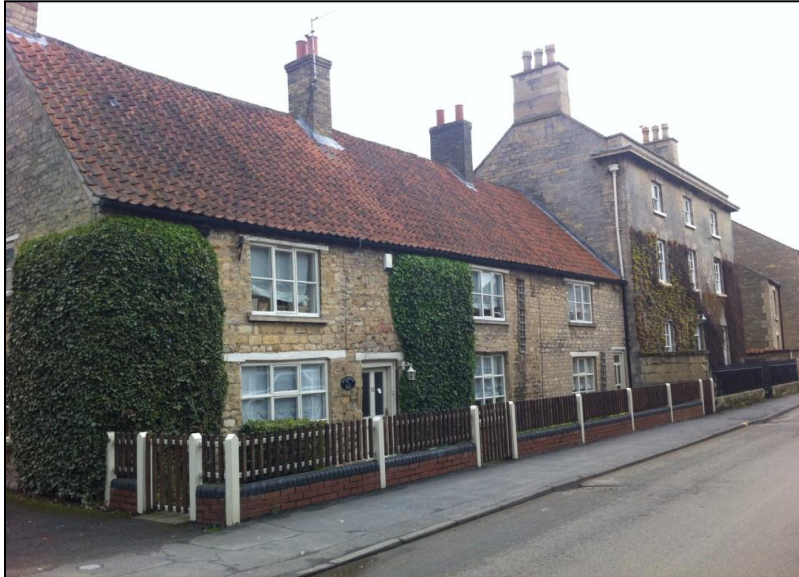
Fig.2 The natural palette of materials and traditional construction methods confers harmony in the streetscene as at The C17th Wheelwrights (long low range) and No.8 High Street. Both buildings are Grade II listed.
