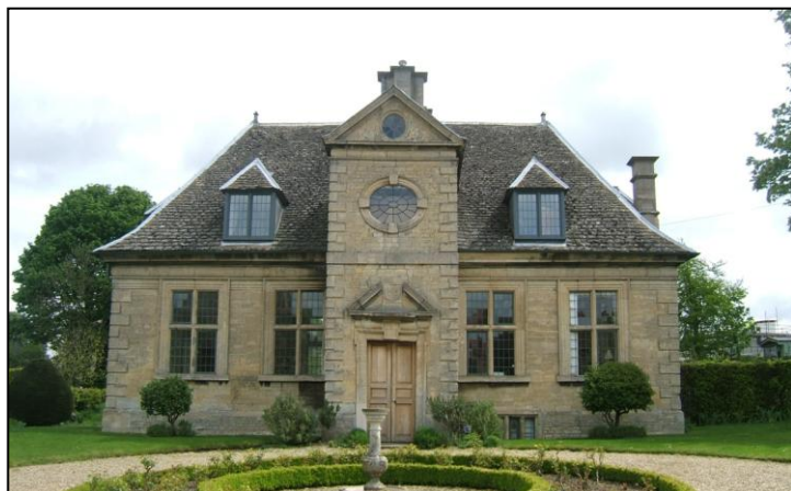
Fig.5 The Grade I listed Willoughby Library and Art Gallery is of exceptional interest and stands prominently within the conservation area at the top of Morley's Lane.
